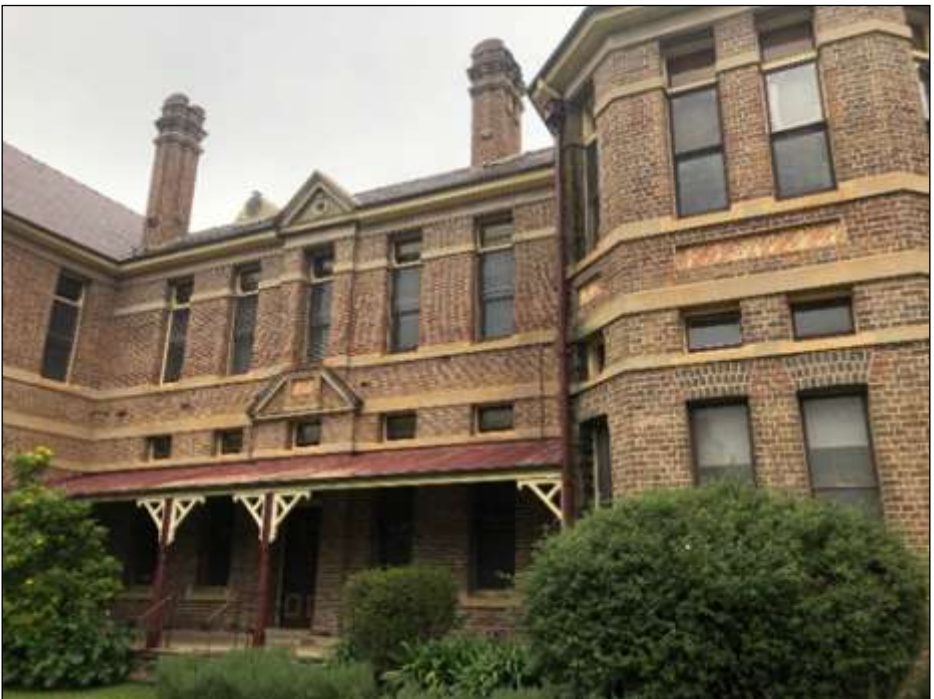
Carrington Hospital here illustrating the windows that were crucial for ventilation. (G Jeremy)
